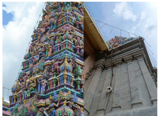
Figure 9: A Photograph of the ESE air termination system installed close to the entrance gate and well below the top of the structures in the close vicinity.
