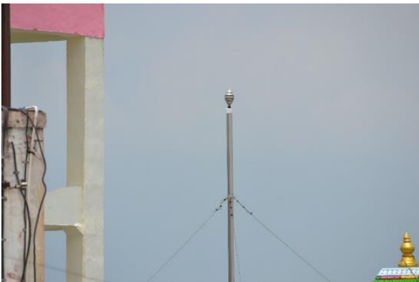
Figure 9: A Photograph of the ESE air termination system installed close to the entrance gate and well below the top of the structures in the close vicinity.
